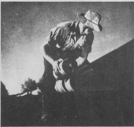
16 After welders had joined 200-foot lengths of eight-inch pipe, mechanical trench diggers prepared a channel along a surveyed course. Here pipe is being insulated to protect it
